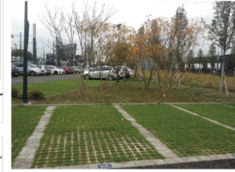
Un parking drainant
